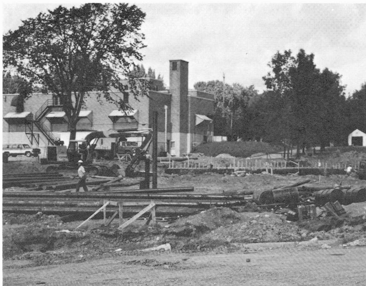
Pile-driving for a new extension to the complex which will house Forest Pest Management Institute staff: the old Insect Pathology Research Institute in the background will be demolished when this new building is completed.
